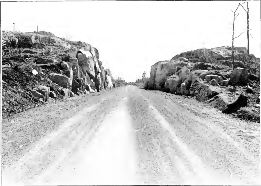
Rock Cut, Highway No. 7, Eight Miles East of Marmora.
